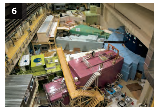
MLF Experimental Hall The neutron beamlines covered with the radiation shields extend from the deep blue neutron target station in the light center of the photo to lower left.
