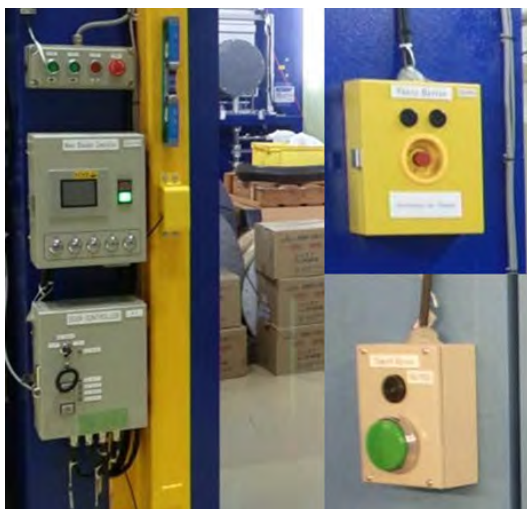
Figure 6. PPS devices at the H1 area: entrance door (left), panic button (top right) and search button (bottom right).
