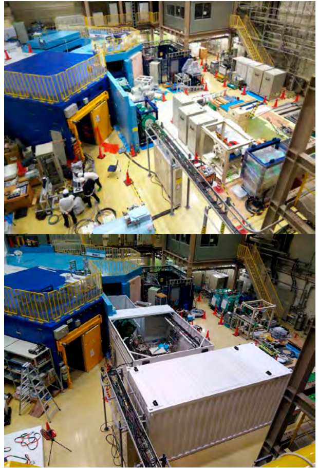
Figure 4. Experimental hall No.1 before (upper) and after (lower) the construction. The roofs of the S2 area are temporary removed.
