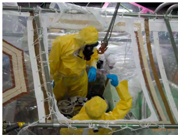
Figure 2. A snapshot of the MUSE target team working on the target replacement assembly, where the radiation workers wearing airtight suits are in a temporary greenhouse to contain radioactive contaminants.
