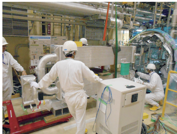
Figure 2. Taking out the heat exchangers from the cold-box.
