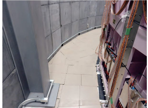
Figure 3. The floor is covered with tiles of B_4C (1 cm thickness). The upper surface of tiles are covered with flooring material.
