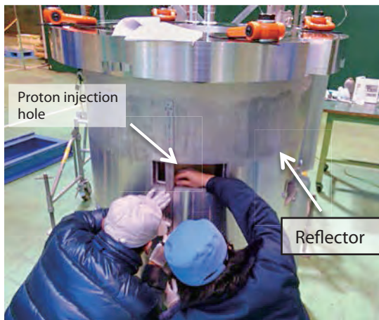
Figure 3. Dimensional check of reflector fabrication.
