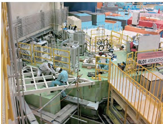
Figure 3. The extension floor under construction.
