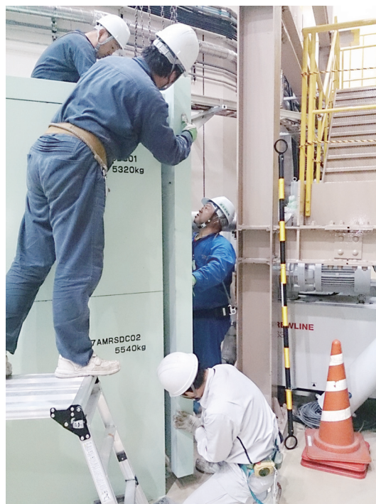
Figure 3. Additional shielding on the beam dump of AMATERAS.
