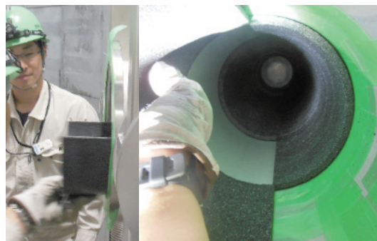
Figure 2. B 4 C liners (10 mm in the thickness) were inserted in-side the get-lost tube of AMATERAS.
