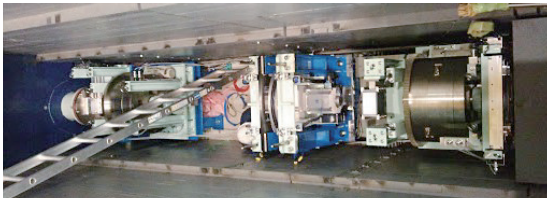
Figure 2. Optical devices inside the preposition shield tunnel.
