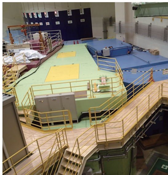
Figure 1. External view of the beam line shielding.
