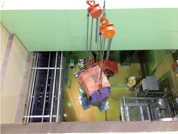
Installation of octupole magnet from M1 tunnel.
