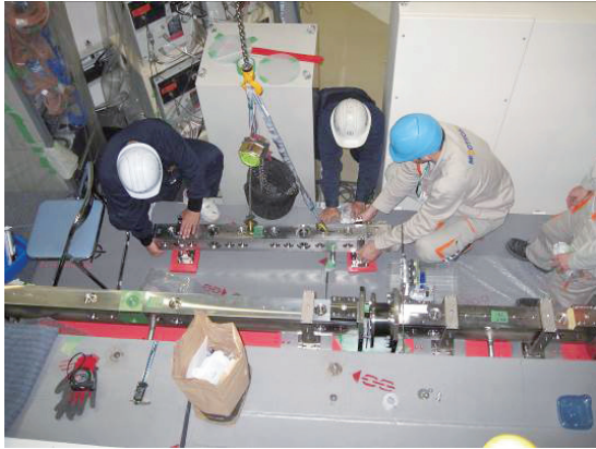
Figure 4. Re-alignment of AMATERAS beam-transport.
