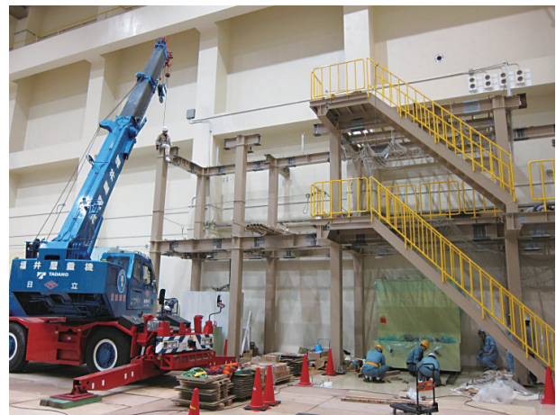
Figure 2. Construction of the power supply yard.
