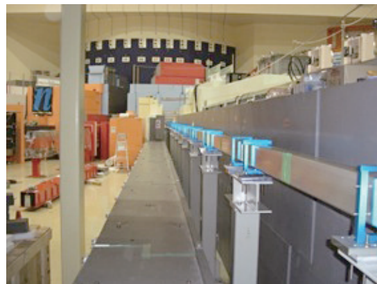
Figure 1. New aluminum vacuum jackets. One unit is about 2 m in length and a support pillar is installed in each unit.
