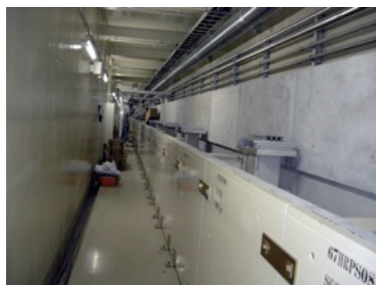
Figure 2. New design of the beam line shield of the straight guide section. Concrete containing boron is used.
