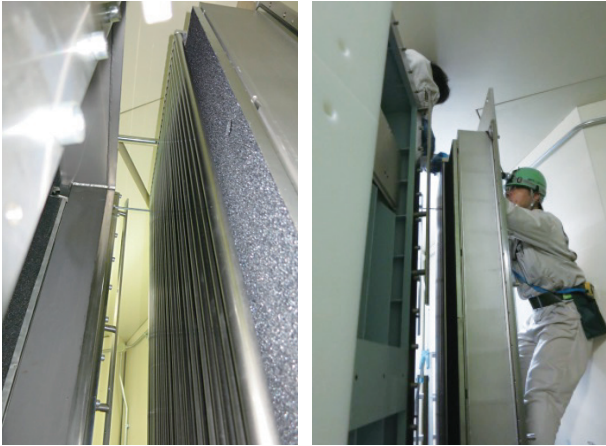
Figure 2. Installation of the detectors by the technical support staffs of MLF.
