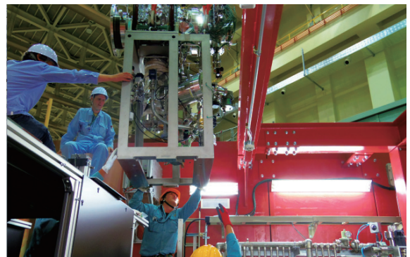
Patrick Strasser and Yutaka Ikedo work with contractor technicians on the Mu production chamber in the U1A area.
