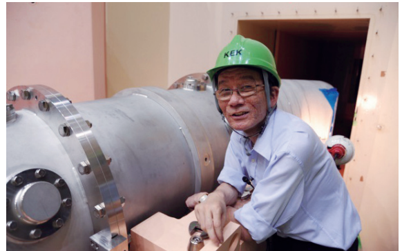
Koichiro Shimomura with the SuperOmega curved soleoid installed at the U-line – the world's highest intensity surface muon channel.
