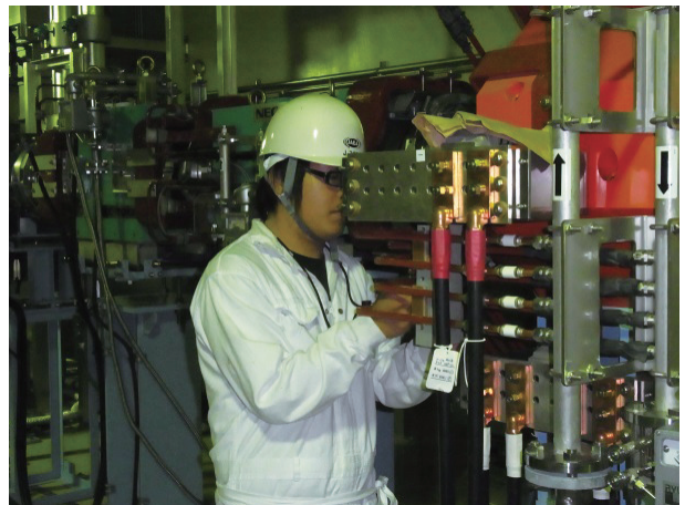
Maintenance work is carried out on the water channel of the quadrupole magnets of the proton beam transport system.
