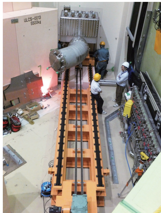
Figure 3. The curved solenoid was set proper position. A part of linear guide at the experimental area was also shown.
