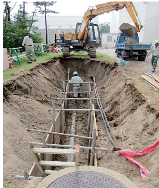
Figure 2. Restoration work for a drain pipe.
