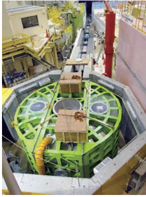
Figure 4. The installation of the DNA vacuum chamber. (October 13, 2011)
