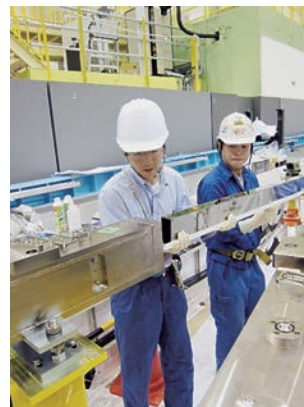
Figure 1. The insertion of a super mirror guide into a metal jacket. (October 22, 2011)
