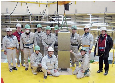
Figure 5. The installation of analyzer crystal units. (January 06, 2012)
