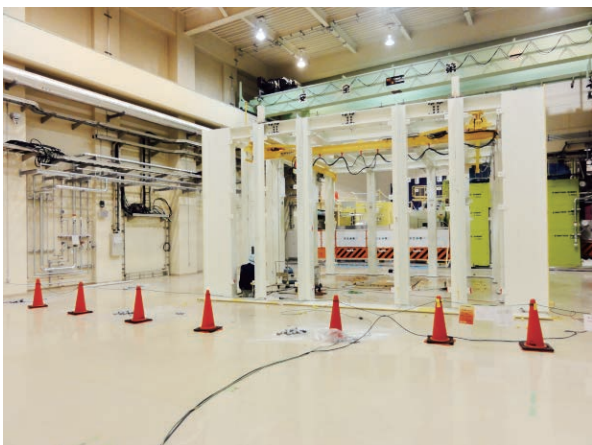
Figure 3. Floor of the west-side extension building after removal of shields and diffractometers of BL18 and BL19.
