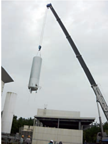
Figure 3. Temporarily removing the helium buffer tank.
