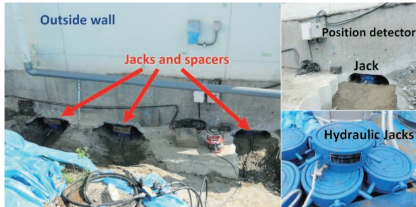
Figure 5. Jacking the extension building up by many hydraulic jacks.
