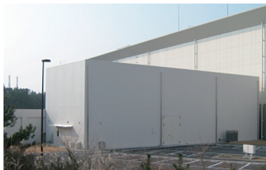
Figure 2. The view of the experiment building of BL09 (SPICA).
