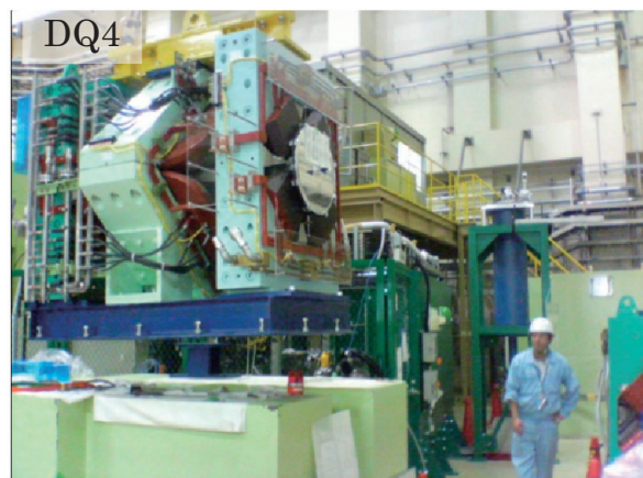
Figure 1. DQ456 triplet installation.
