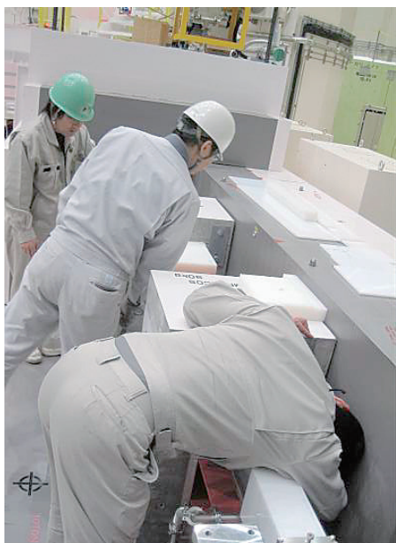
Figure 5. Installation of polyethylene blocks at the beam line.
