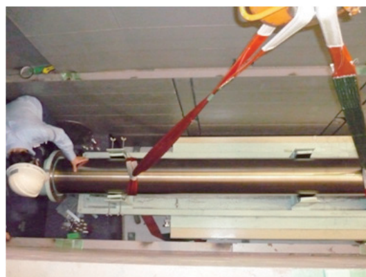
Figure 1. The insertion of a super mirror guide into the biological radiation shield on BL02.(July 16, 2010).
