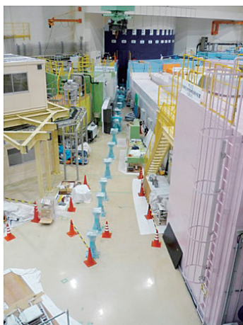
Figure 3. The installation of the struts for mounting super-mirror guide tubes and disk chopper. (August 31, 2010).
