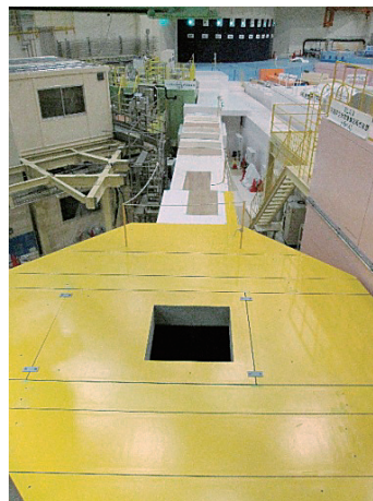
Figure 5. The installation of radiation shields for the DNA vacuum chamber. (February 19, 2011).
