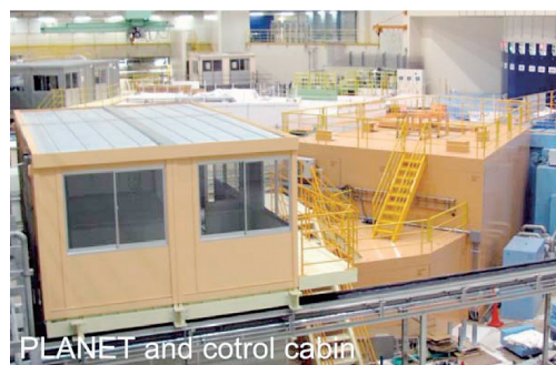
Figure 1. PLANET and the control cabin.
