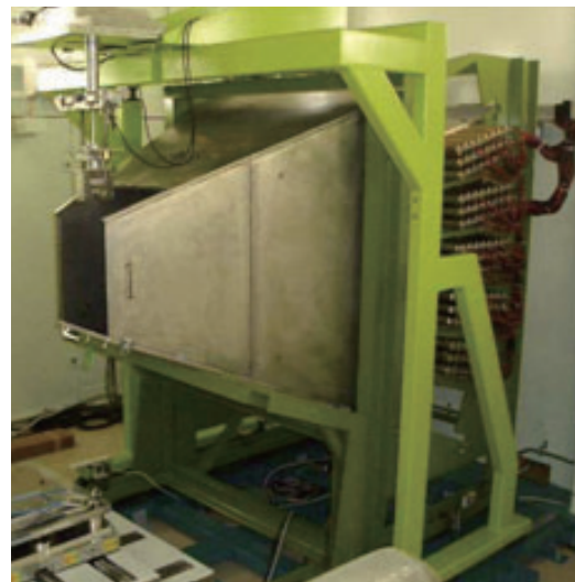
Fig.4 Detectors installed at the south bank of TAKUMI
