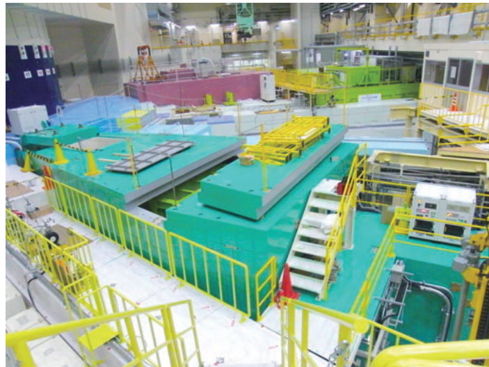
BL15 being under construction.
