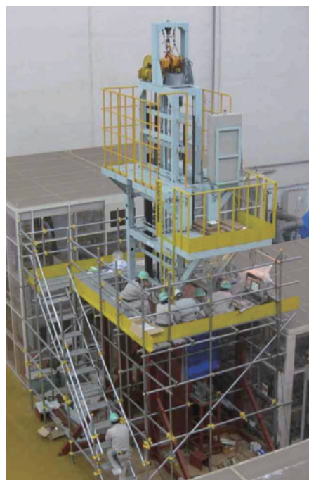
Fig.2 Core-vessel insert handling devise in testing in the HENDEL building
