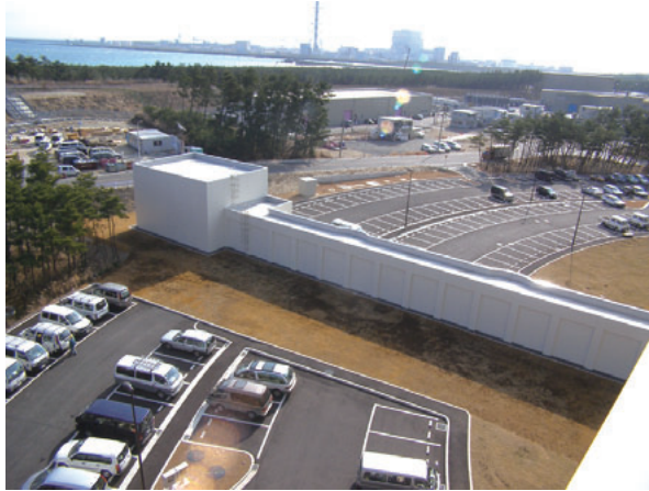
Fig.1 The east building for BL08 (SuperHRPD).
