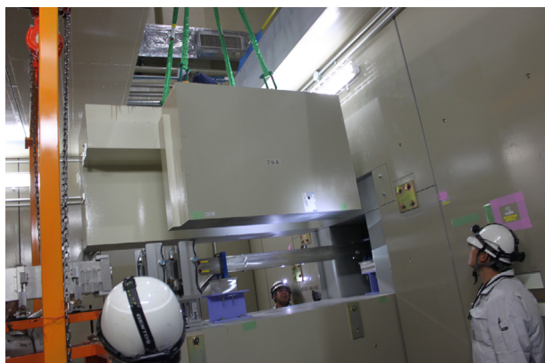
Figure 3. The work scenery of removing the concrete blocks for radiation shielding around the end of the supermirror guide of SPICA.
