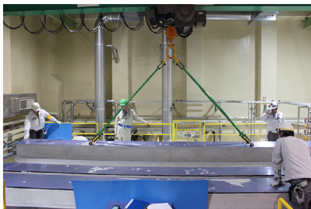
Figure 2. The work scenery of removing the concrete blocks for radiation shielding located at the top of the main body of SPICA.
